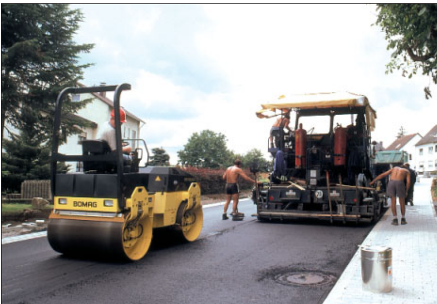
BW 138 AD, the powerful performer directly behind the road finisher.
